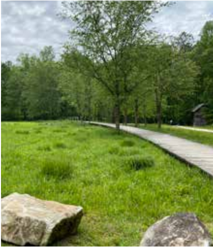
FIGURE 7.2. The community biological wastewater treatment at Serenbe in Chattahoochee Hills, Georgia, appears to residents and passersby as a field among forests. © Catherine O. Ryan
